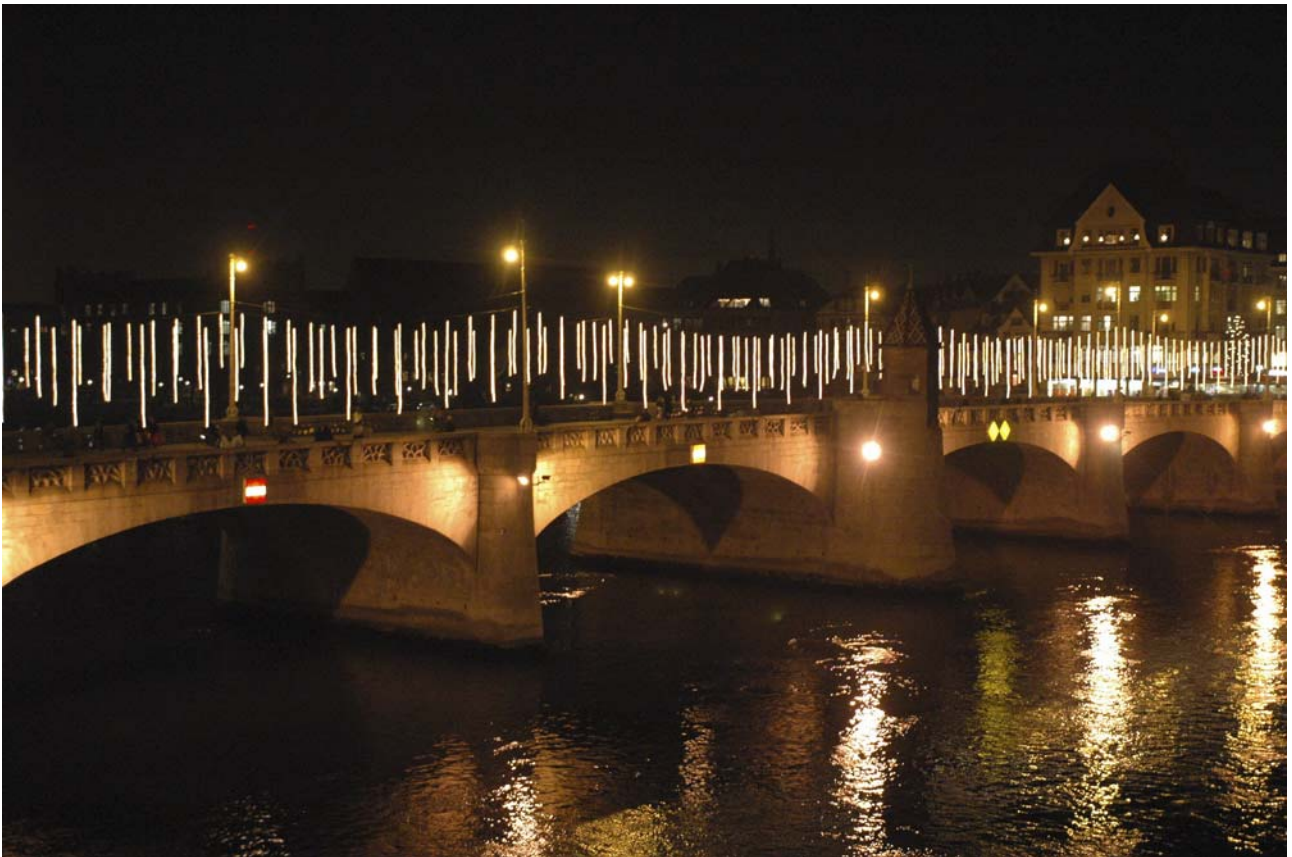
The Basler "Middle" Bridge, over the river Rhine, with foundations from the 13 th century
